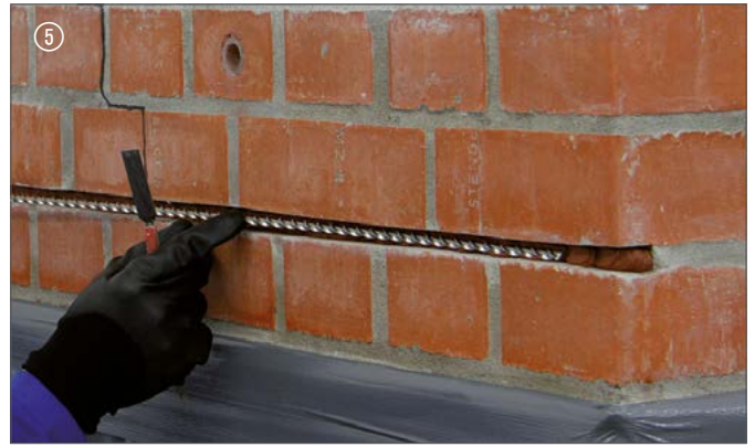
5 Spiralanker setzen | Place the spiral anchor
