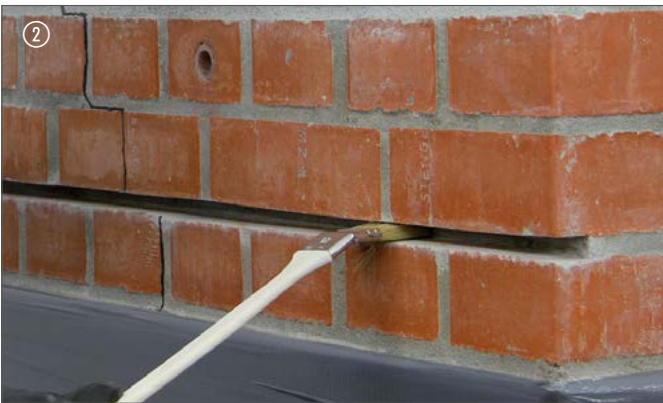
2 Fuge reinigen | Clean the joint/slot
