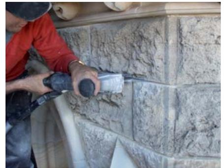
The AS200X Brick and Mortar Saw offers extraordinary control and precision and allows efficient and low dust cutting up to a cutting depth of 170 mm (with the XL General purpose blades, No. 000-03-297). This makes the AS200X Brick and Mortar Saw the ideal cutting tool for various applications, e. g.
