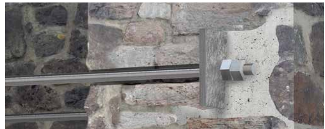
Fig. 3 Anchor plate detail
