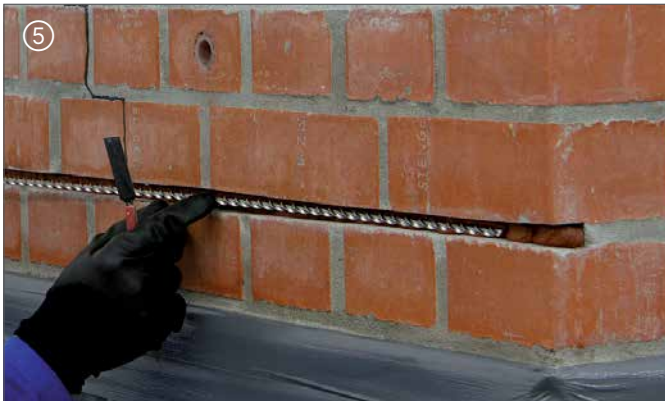
⑤ Spiralanker setzen | Place the spiral anchor
