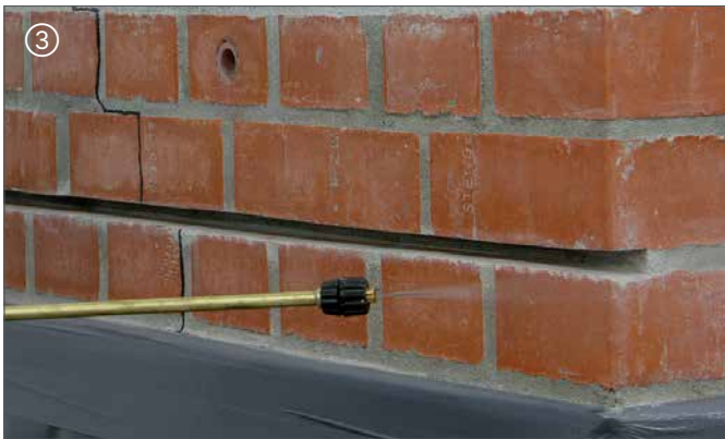
③ Fuge vornässen | Wet the joint / slot
