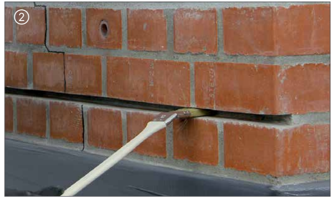
② Fuge reinigen | Clean the joint / slot
